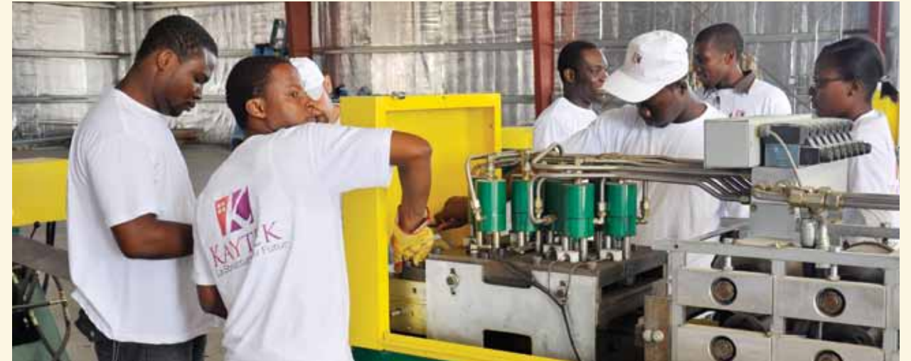
Employees at GaMa's KayTek factory produce steel framing for construction.
