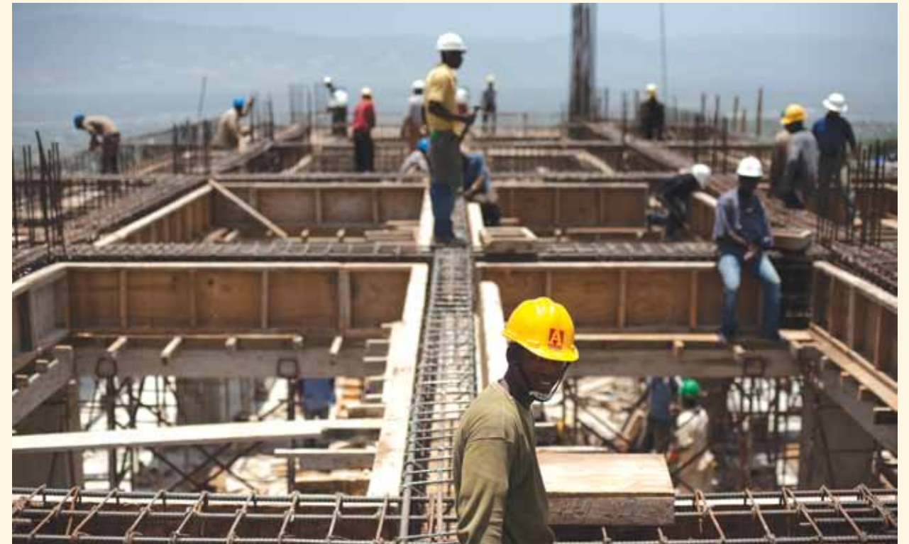
Construction workers add floors to the Royal Oasis Hotel.
